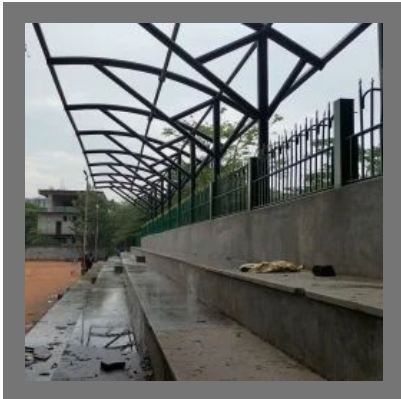
Outdoor Shade Structure Fabrication Service
